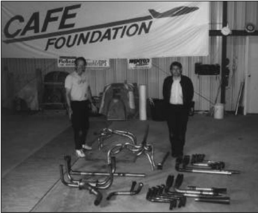
**Brien Seeley, left, and Ed Vetter with several of the exhaust pipe models which will be undergoing testing. The pipes are adjustable for both header and collector length and diameter. The stock Mooney system is at lower left.**
